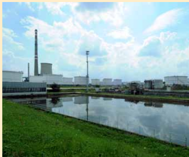
Sewage treatment plant in the Kralupy nad Vltavou refinery
